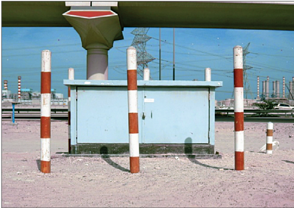
1.4.4 Vertical mounted link box with steel bollard protection
