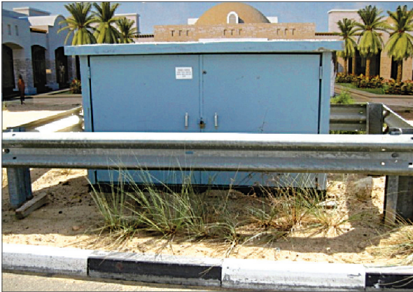
1.4.5 Vertical mounted link box with steel crash barrier protection on the side of a road.
