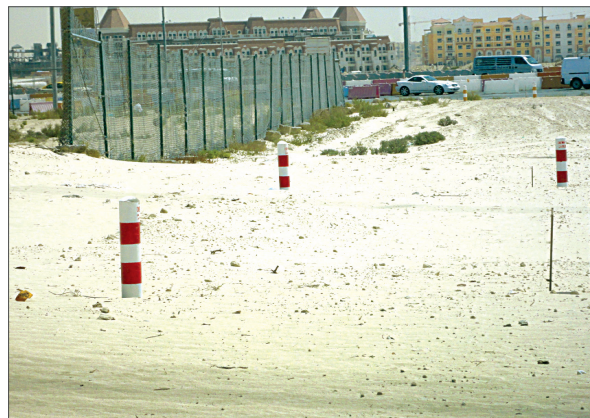
Location of 132kV cable Joint bay installation with identification route marker
