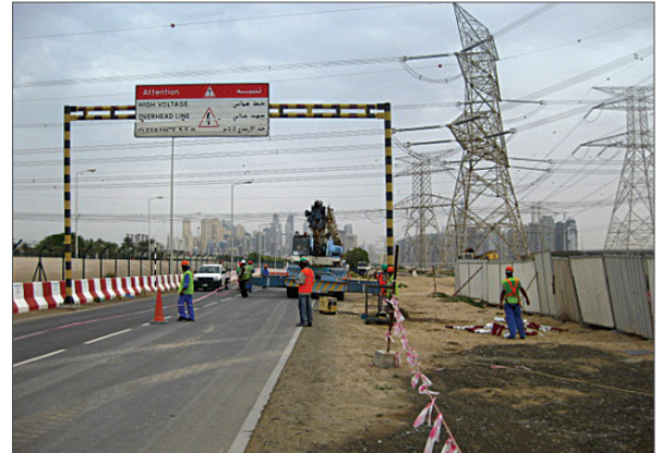
1.4.8 Permanent-height-limit gantry at road crossing
