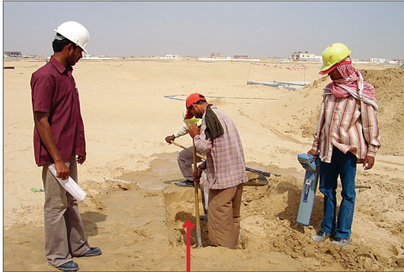
Locating the service by referring the NOC
