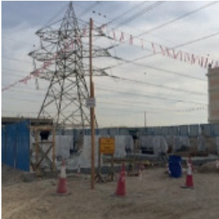
Clearance confirmed & Height limit gantry provided
