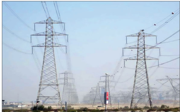
d. 132kV Steel Lattice (Double Circuit Tower)
