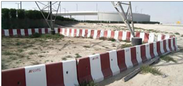
Tower foundation protected with concrete barrier
