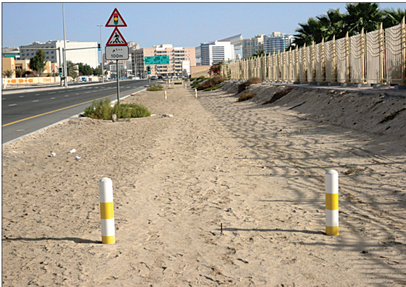
1.4.6 Surface-pole-type route markers installed at 50-metre intervals.
