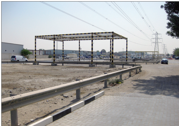
1.4.9 Permanent height-limit gantry at a road crossing
