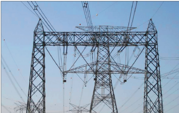
c. 400/132kV Gantry Tower
