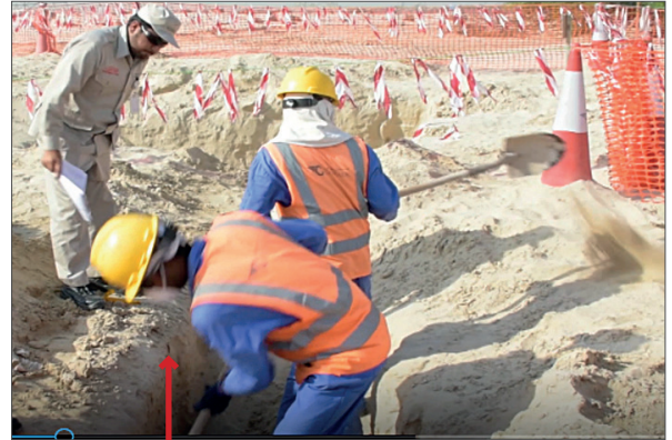
Manual excavation for trial pit to trace the service
