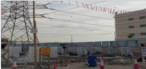
Tower foundation protected with concrete barrier
