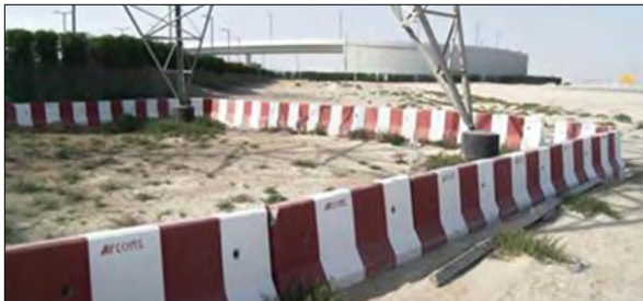
Tower foundation protected with concrete barrier
