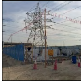
2.3.b Clearance confirmed & Height limit gantry provided
