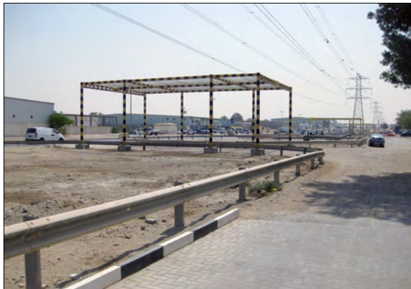
1.4.7B Permanent height-limit gantry at a road crossing
