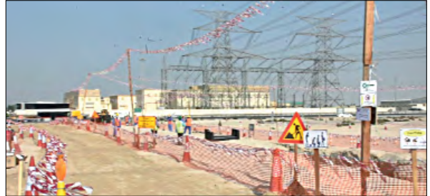
Vehicle movement restricted near transmission lines
