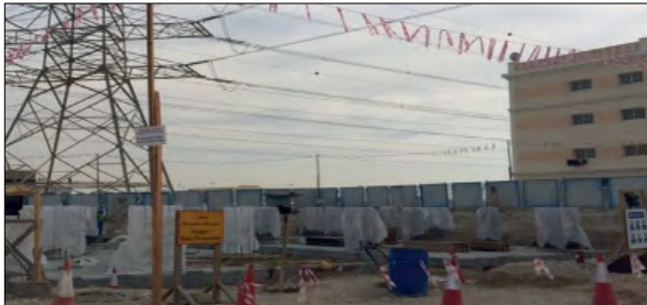
Tower foundation protected with concrete barrier
