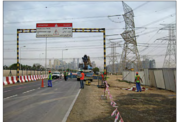
1.4.7A Permanent-height-limit gantry at road crossing
