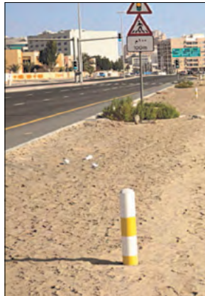
1.4.4A Surface-pole-type route markers installed at 100-metre intervals.
