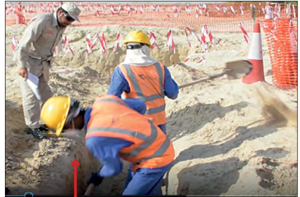
Fig 3.1.3 Manual excavation for Trial Pit.
