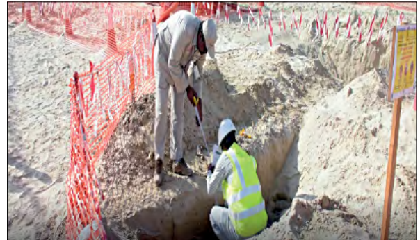
Fig 3.1.4 Trial pit verification.
