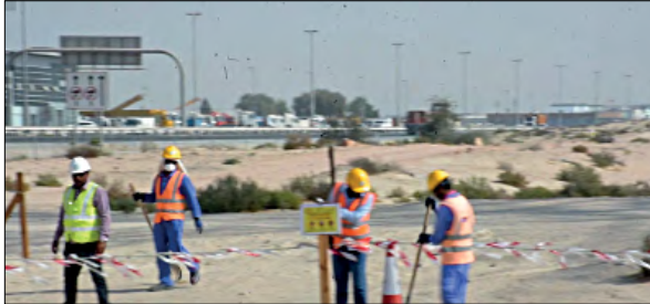
Identifying and installing barricades and signs
