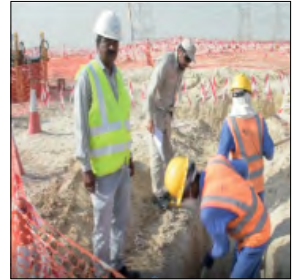
2.3.c Manual excavation
