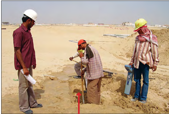
Fig 3.1.2 Locating 132kV cable through Trial Pit.
