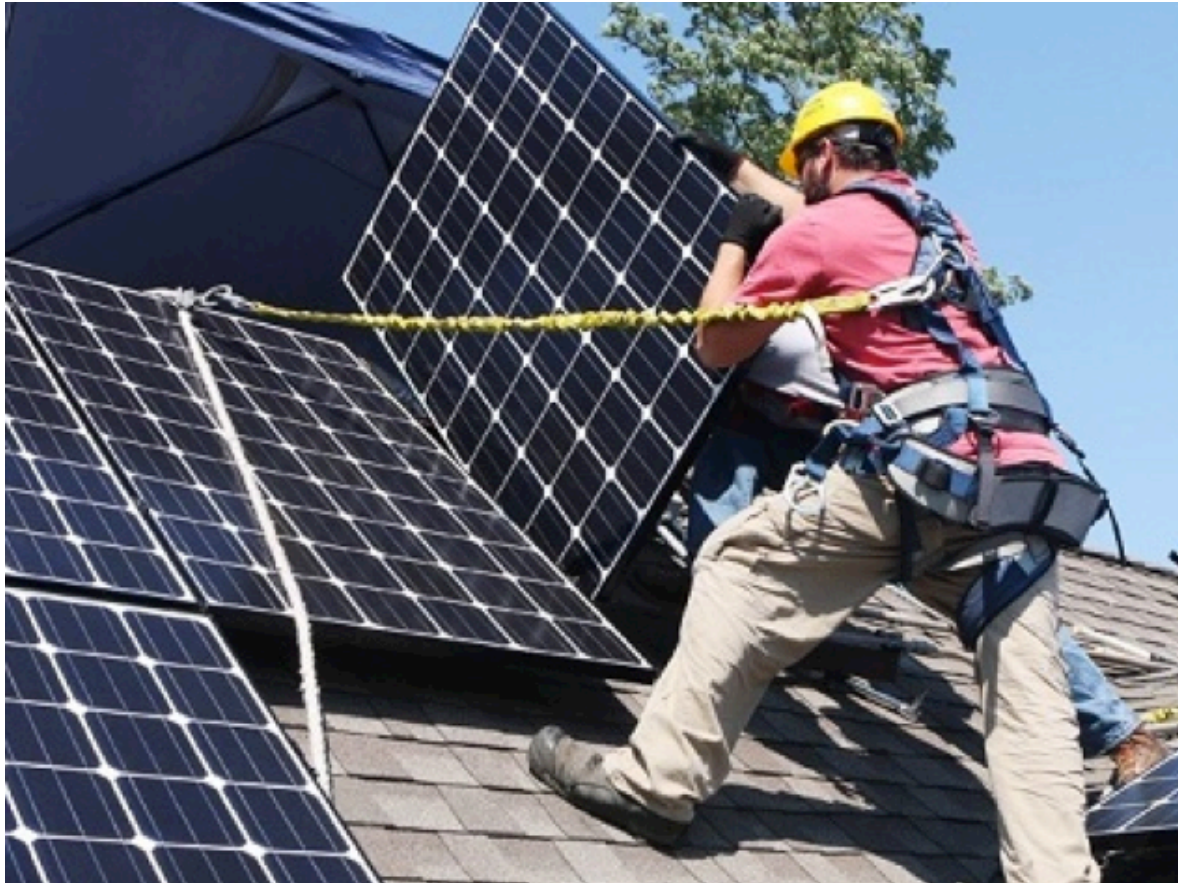
Figure 3 – Example of installation of a PV system in presence of several risks
