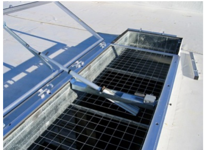
Figure 4 – Example of safety nets installed below skylights
