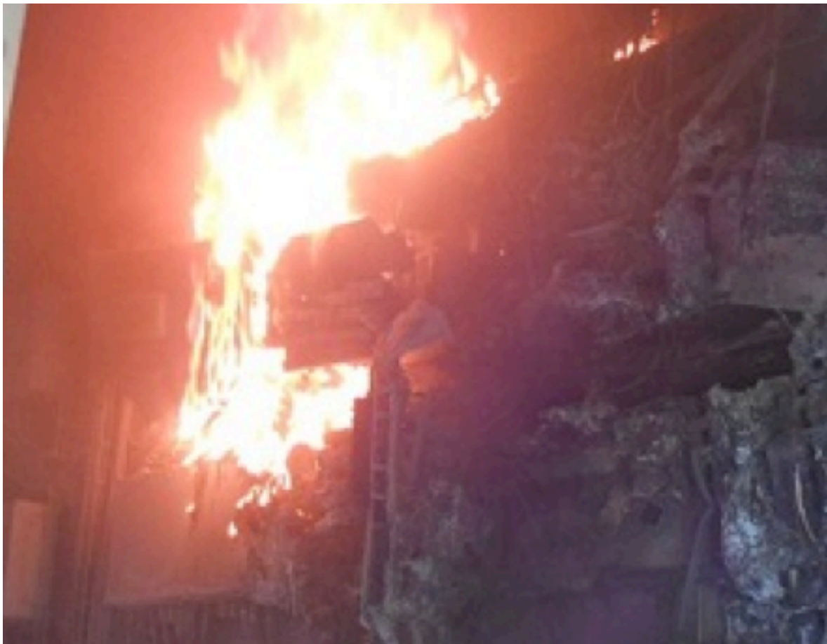
Figure 8 – Example of combiner boxes burning despite fire fighting operations, because they are still fed by the PV array
