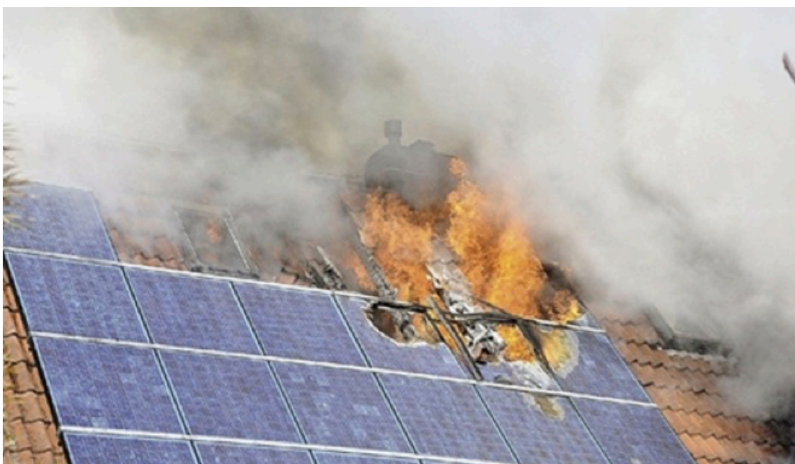
Figure 6 – Example of effects of a fire in a PV system - that originated in combiner boxes
