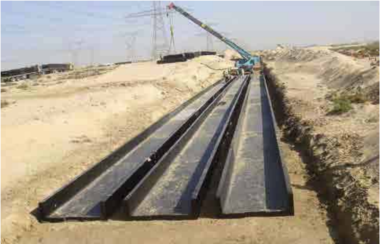
Photo: 132 kV Trough Laying
