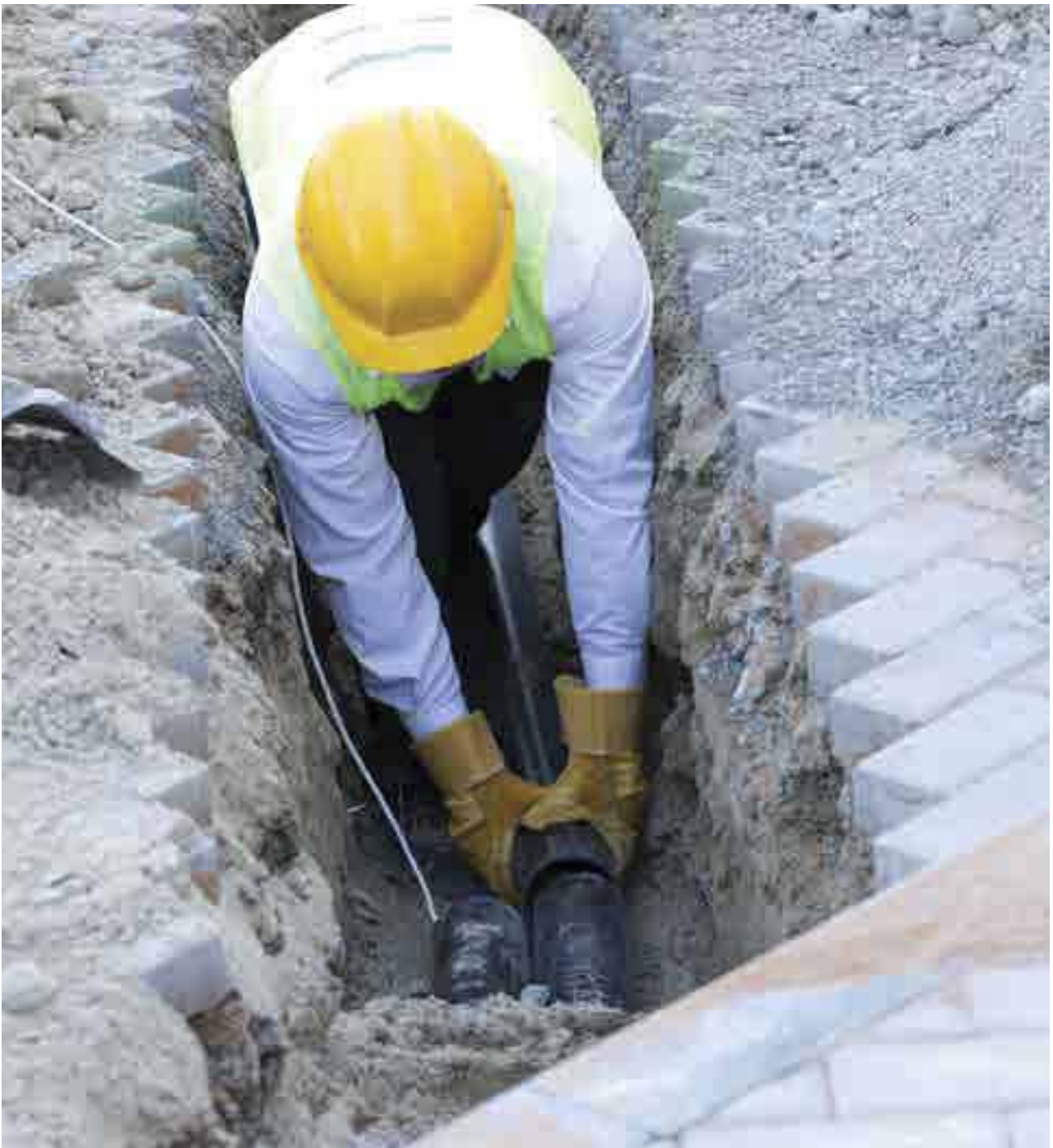
Proposed DEWA Electrical Ducts, Extension and protection of existing Ducts
