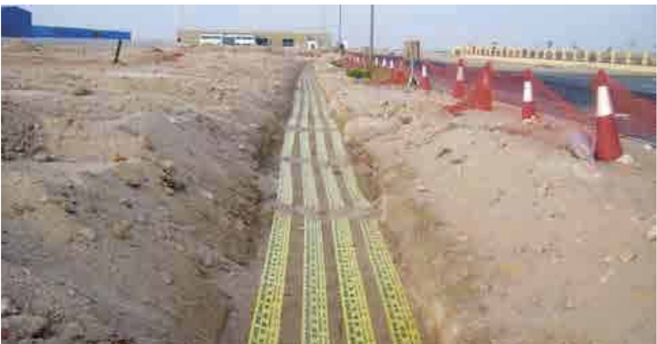
Laying of High Voltage (HV) Cables: Site Photos
