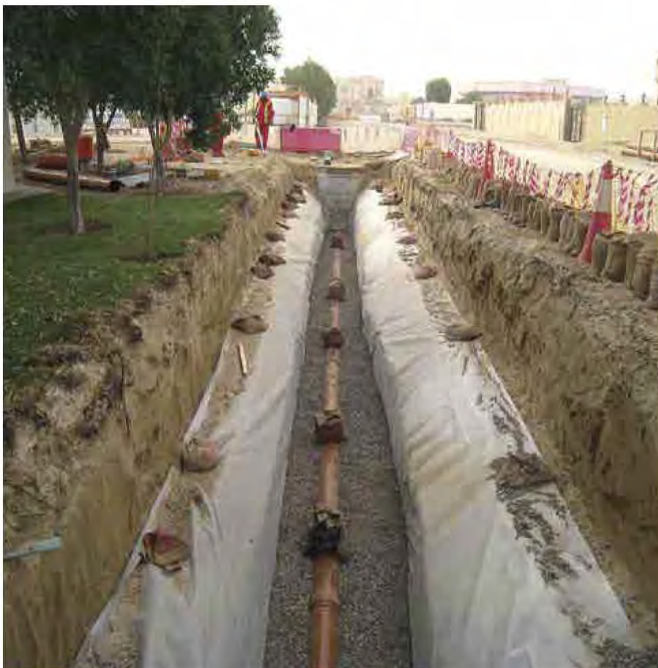
Laying of Drainage Gravity pipeline
