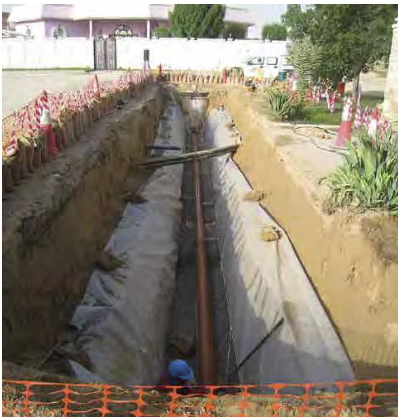
Laying Sewerage Gravity line
