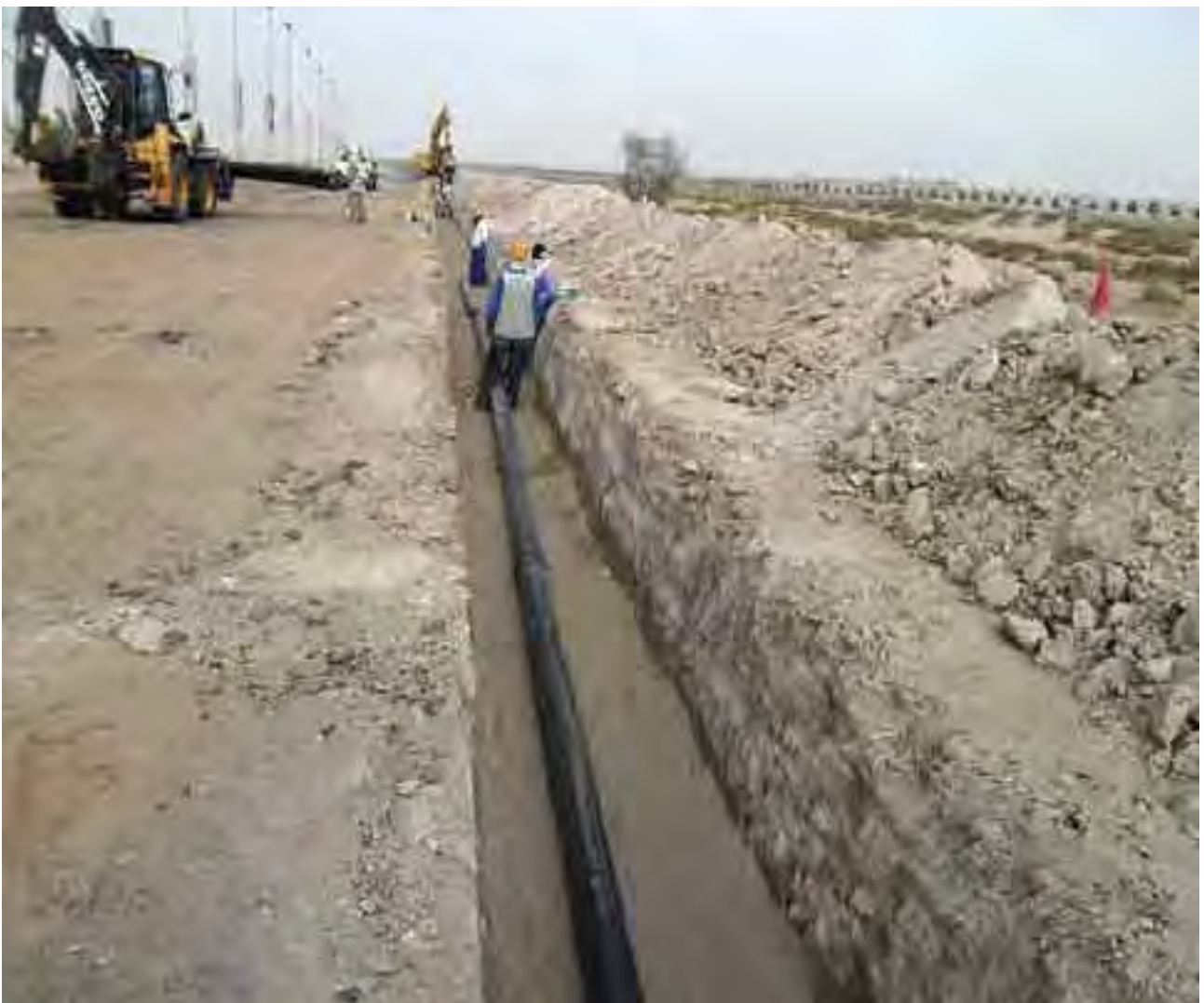
Laying Irrigation Distribution Network
