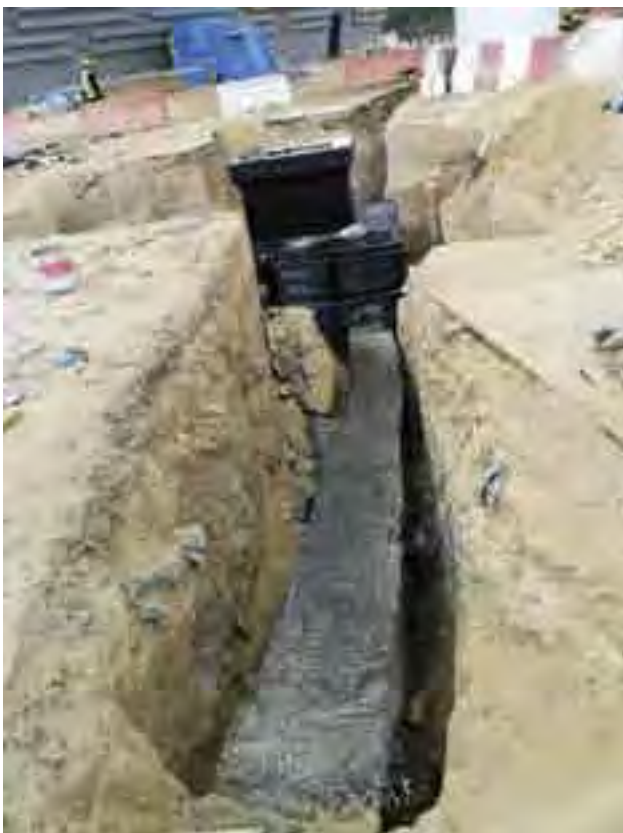
Photo: Telecommunication ducts.
