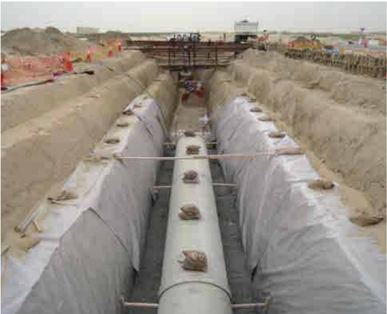
Laying of Sewerage Pipeline
