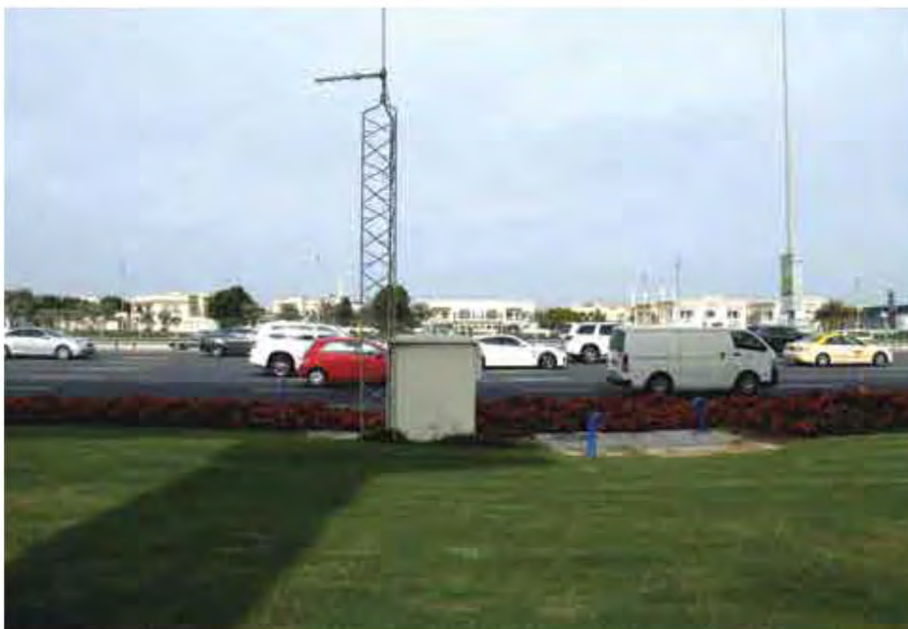
Transmission Water Line with Valve chamber, RTU and Antenna.
