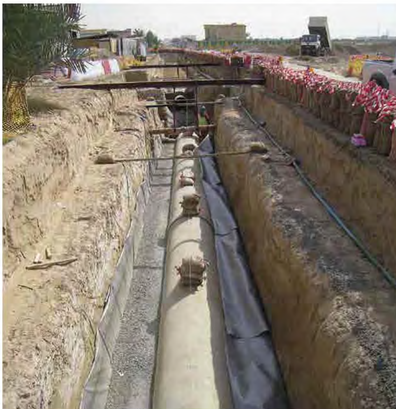
Laying of Drainage Pressure line
