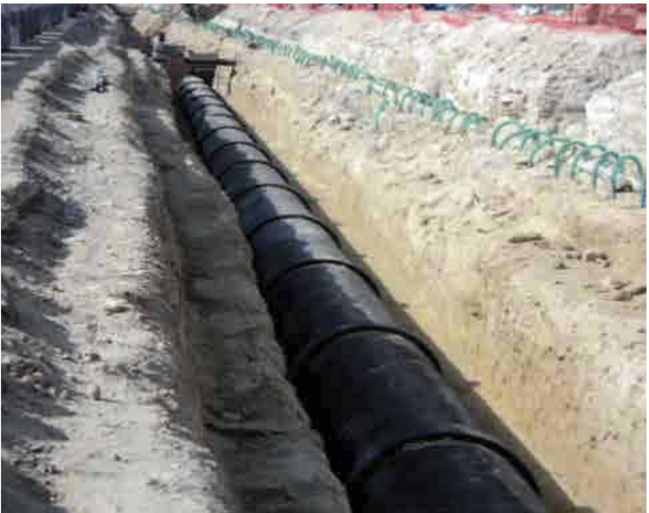
Laying of Irrigation Main Network
