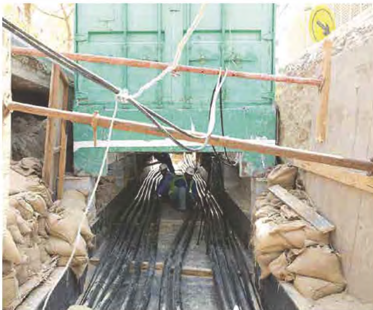
Laying of Proposed Utilities - Electricity 132 kV Joint Bay/Transition Joint
