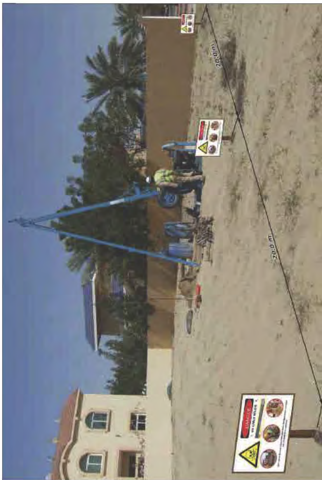
Photo: 42.1 TEMPORARY WARNING SIGN BOARD INDICATING EXISTING HV SERVICES CLOSE TO PROPOSED SOIL INVESTIGATION LOCATION
