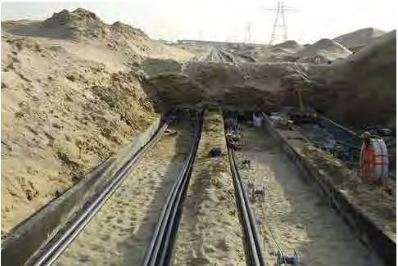
Photo: 132 kV Cable laying inside Trough
