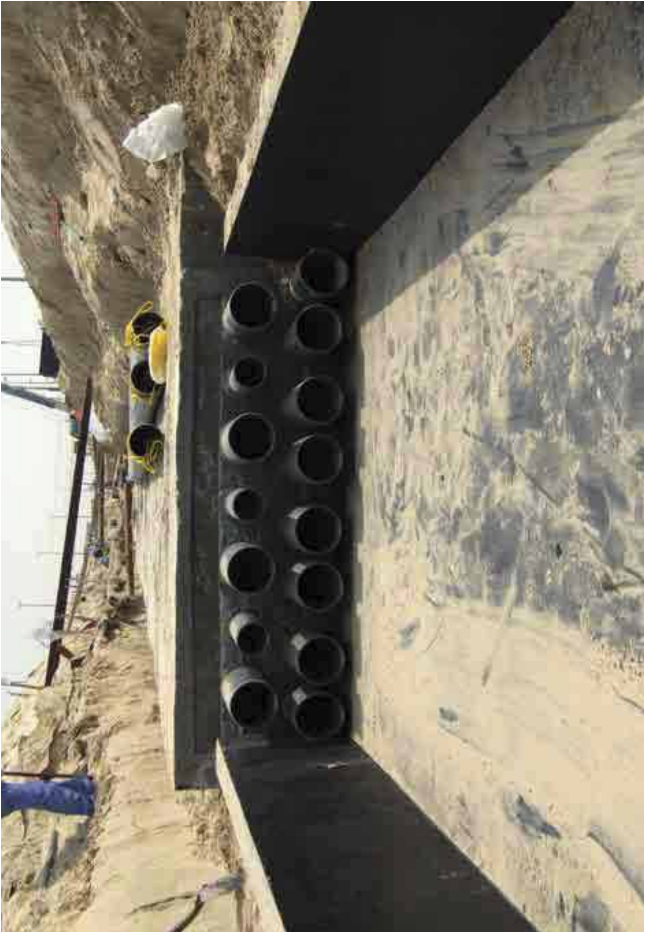
132 kV Duct Bank work at site
