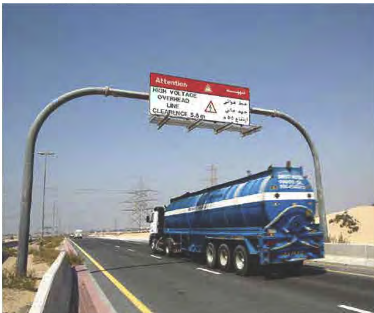
Installation of Proposed Permanent OHL Warning/Head Room Gantry
