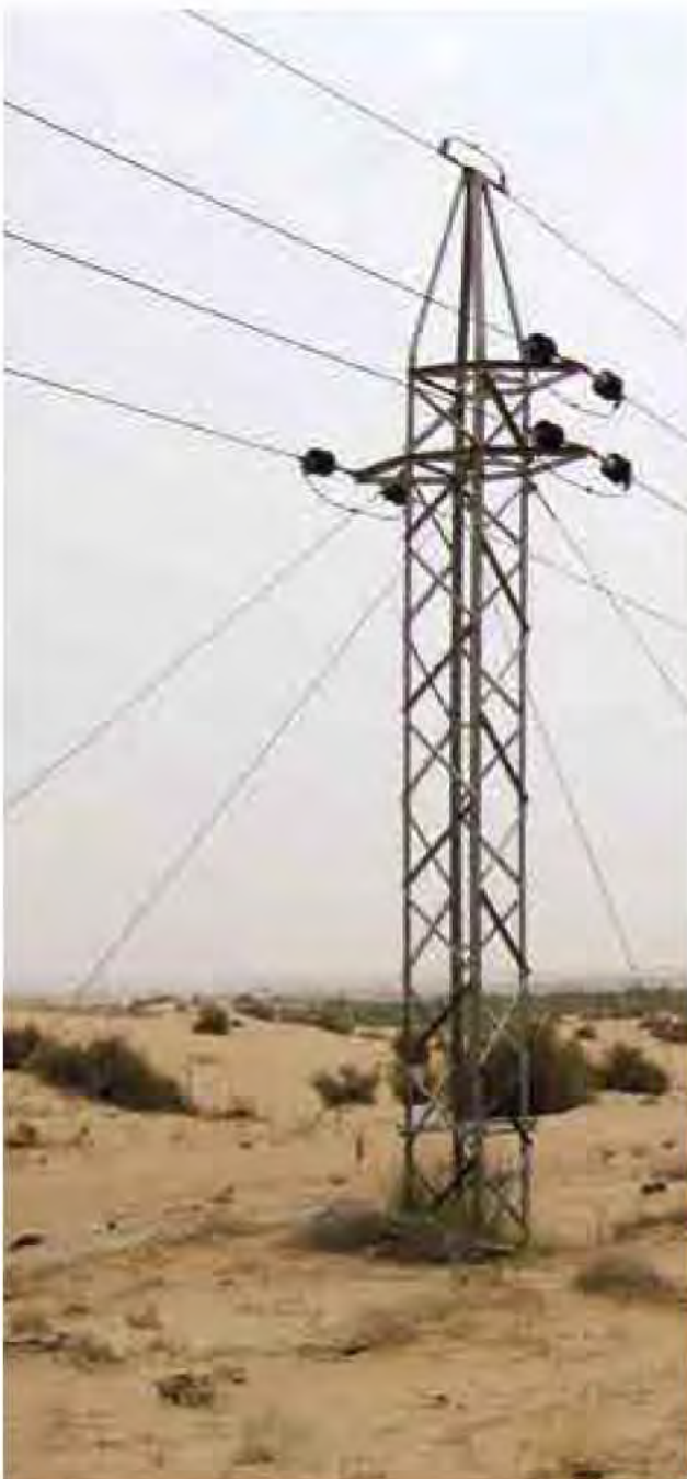
Steel Tower for HV OHL
