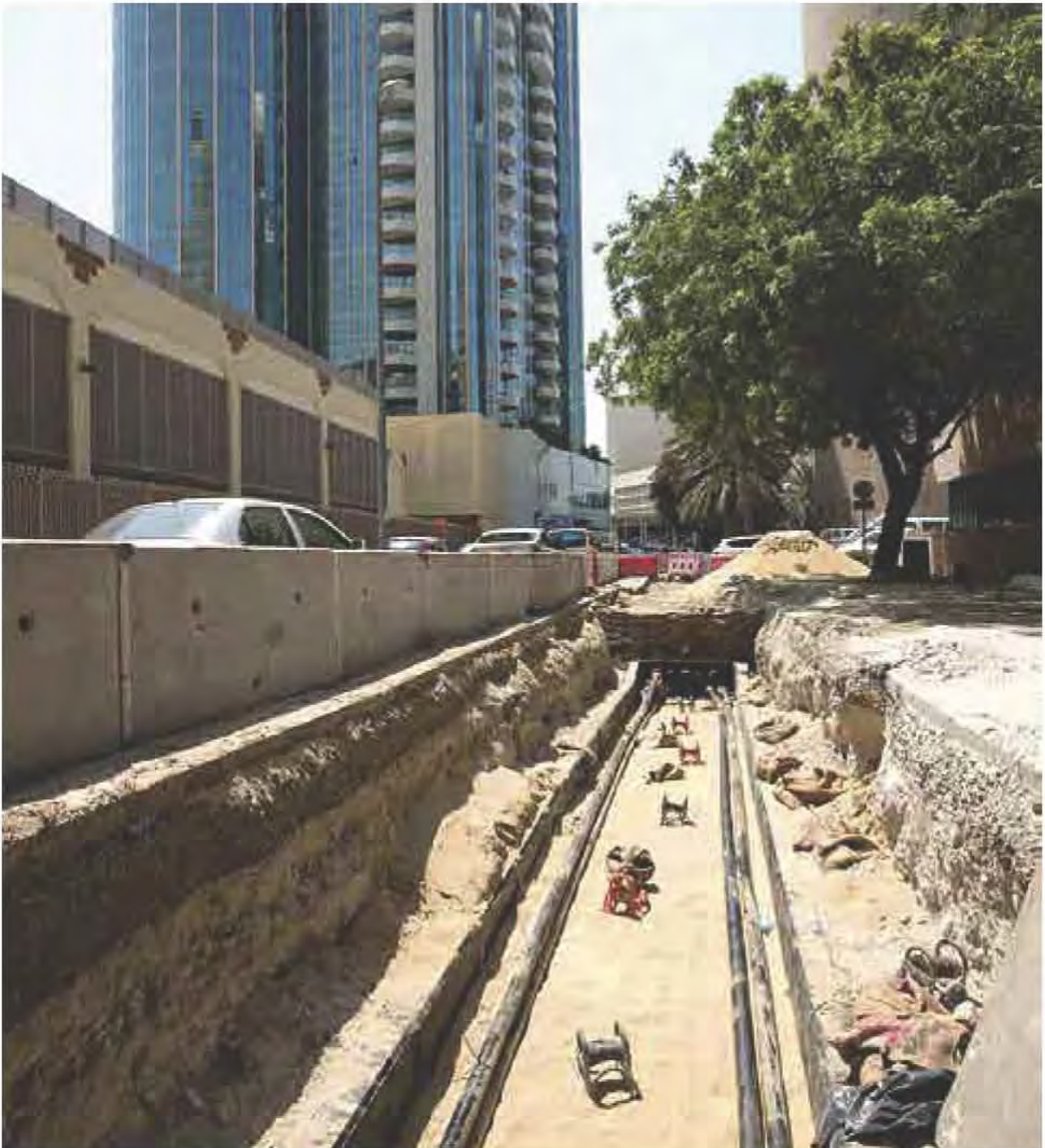
Laying of Proposed Utilities - Electricity 132 kV Duct Bank
