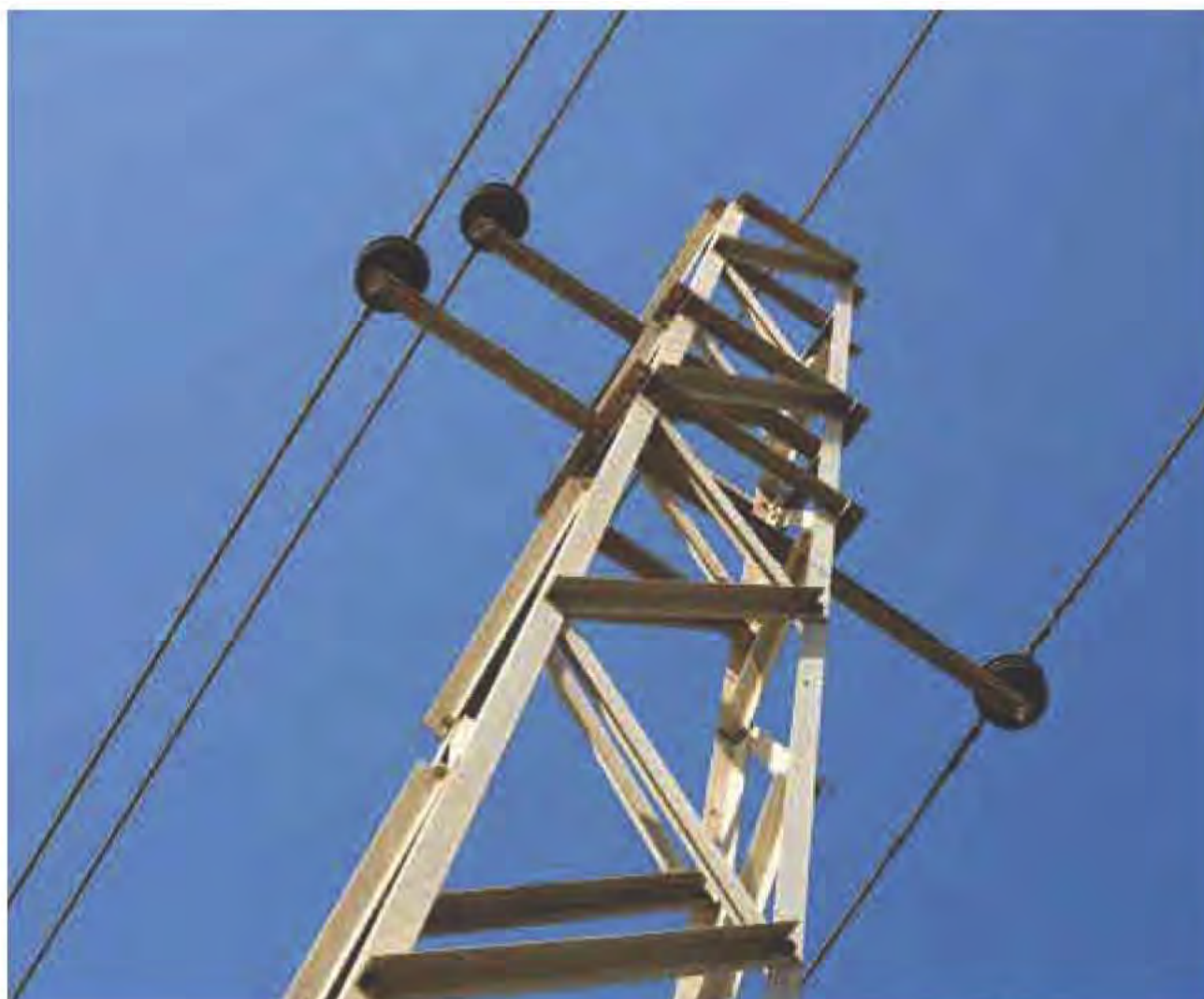
Installation of Proposed OHL - Electricity HV (6.6/11/33 kV)
