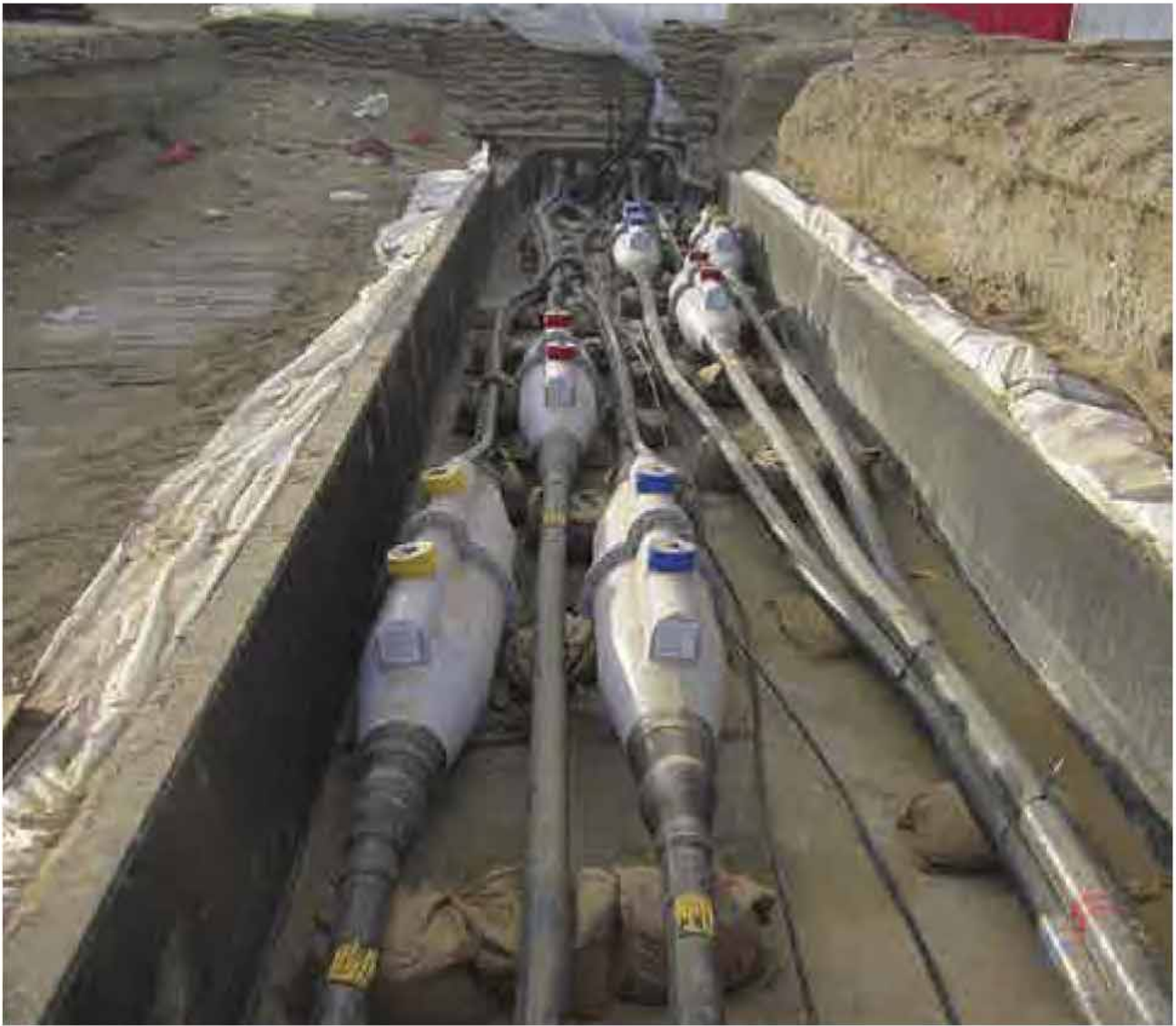
Photo: 132 kV Joint Bay
