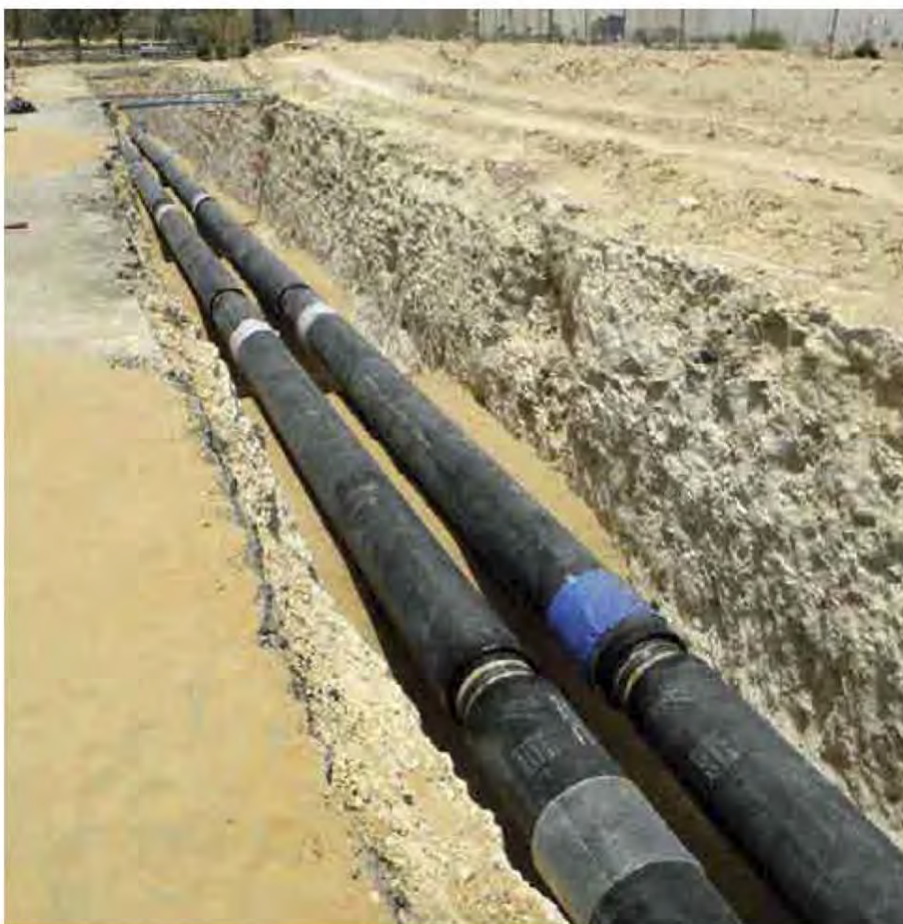
Chilled Water Pipeline.
