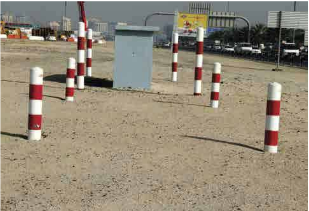
132 kV Joint Bay with Markers and Link Box
