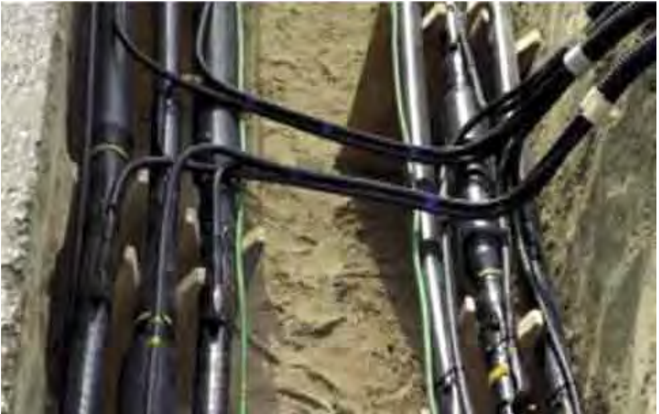
132 kV Link box - Bonding Cable
